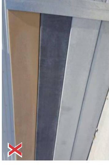
FIGURE 6 - TREATED PINE RETAINING WALL
